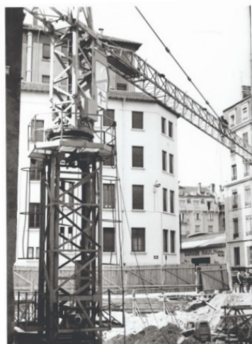
Construction de la MOM © service Archives MOM
